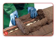
→ Important: Make sure the joints are completely filled with FLEXIM.
