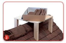
→ Tip: Make a small table to sit FLEXIM strips on to help when working.
