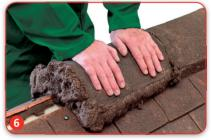
→ Press ridge-cap, with clean hands, firmly down into the centre of the bar, ensuring that FLEXIM is both inside and outside of the ridge-cap. Keep the joints as tight as possible.
