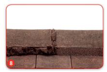
→ A small amount overflowing is ok because you can clean the joints with a finger/spatula.
