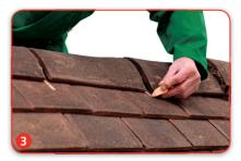
→ Mark the position of the butt-joint with a piece of chalk.
