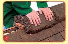
→ Press ridge-cap, with clean hands, firmly down into the centre of the bar, ensuring that FLEXIM is both inside and outside of the ridge-cap.
