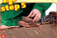
You can use broken tiles (pieces of tiles) to fill up the space under the ridge-cap.
